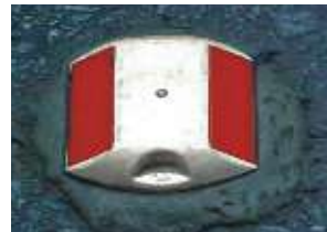
Place the RPM on the thick pack of adhesive without applying excessive pressure
