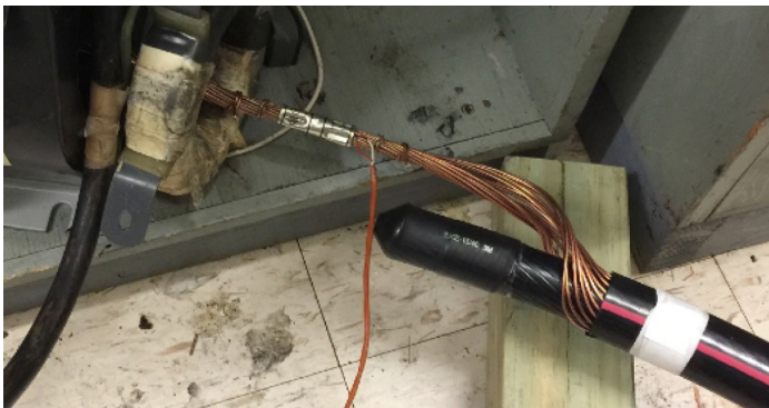
Figure 4: Crimped connector connecting the CN wires. The connector used is a 10006 2/0 CU
