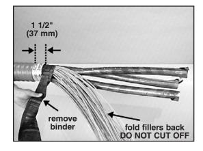
2.3 Cut the phase cores to the appropriate length.
