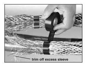
4.9 Connect the ground wire(s) from **Cable X** to the ground wire(s) from **Cable Y**. Make the connection away from the splice bodies.
