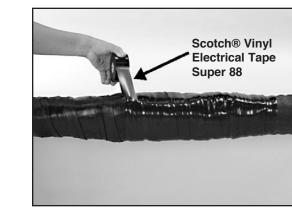
6.6 Cover the applied 3M<sup>™</sup> Scotch-Seal<sup>™</sup> Mastic Tape 2229 with two half lapped layers of Scotch<sup>®</sup> Vinyl Electrical Tape Super 88.
