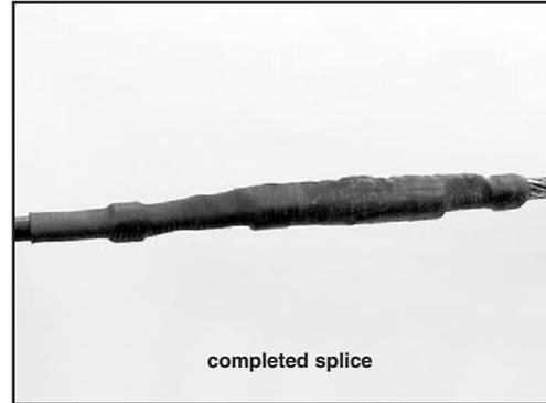
**Note:** *In applications where the splice is regularly exposed to high levels of ultra-violet radiation (i.e. direct sunlight), wrap two half-lapped layers of Scotch™ Super 33+ or Scotch™ Super 88 vinyl tape over the re-jacketing tubes.*
