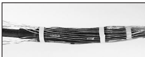
Neutrals straight across splice
