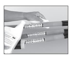
4.5 Apply red compound on cable insulation, making certain to fill in edge of cable semi-cons.
