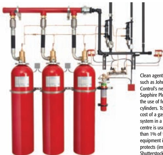
Clean agent systems such as Johnson Control's new 70-bar Sapphire Plus enable the use of fewer cylinders. Top: the cost of a gaseous system in a data centre is usually less than 1% of the equipment it protects (image: Shutterstock).
