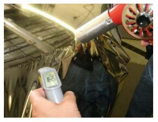
**Figure 2.** Heat the film to 150°F to 180°F (66°C to 82°C) and use an infrared thermometer to monitor the
