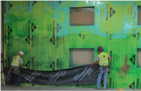
Figure 3: 3M 3015 Installation
