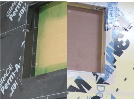
Figure 4: Window Penetration Detail
