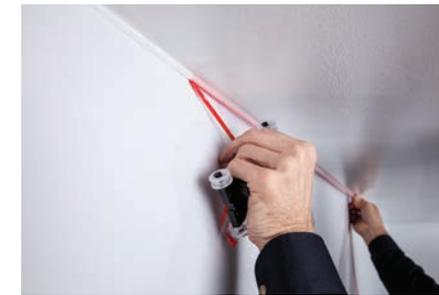
now adapted for the multi-fiber needs of MDU Hallways. The 3M™ Clear Track Hallway Fiber Pathway solution enables fast and easy installation, with minimal disruption for tenants.
