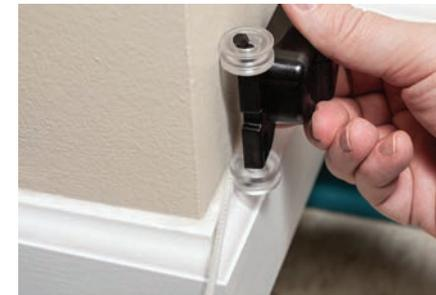
3M™ 900 μm Clear Fiber—ultra bend-insensitive fiber—can be quickly inserted using the handy installation tool. The fiber can then be terminated with a 3M field-mounted mechanical connector or splice.
