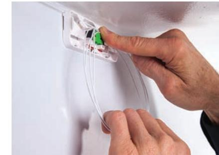
self-adhesive Command™ Strips makes attachment and repositioning easy. The 12-fiber micro-module can then be terminated with a 3M field-mounted mechanical connector or splice for connection to the living unit.
