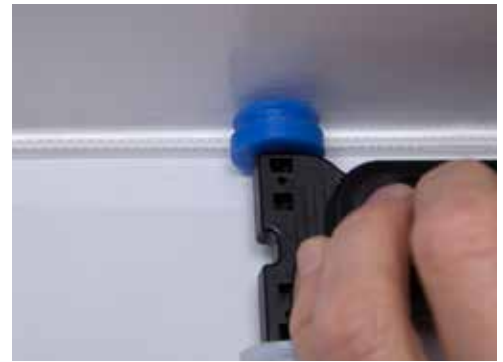
Installation of 3M™ Clear Track 12-Fiber Micro-module into 3M™ Clear Track Hallway Fiber Pathway
