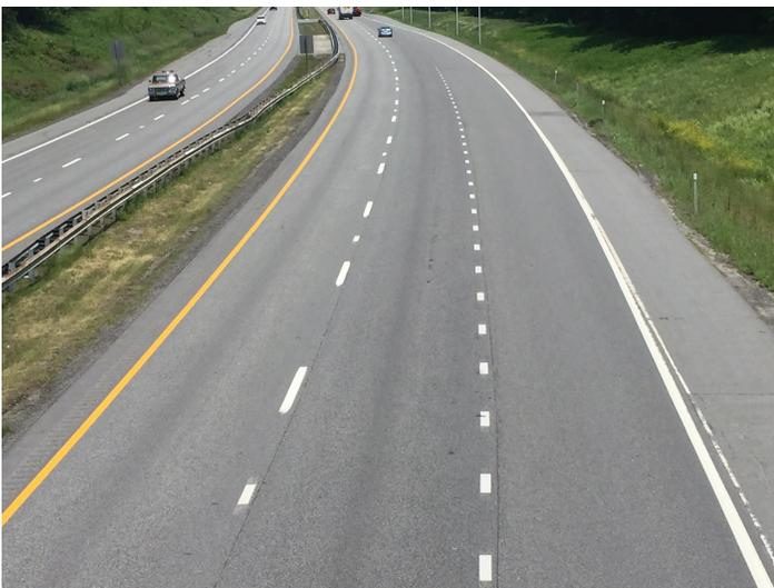
The Maine Turnpike Authority turned to reflective pavement marking tape from 3M after years of using recessed pavement markers that required annual upkeep and maintenance.
