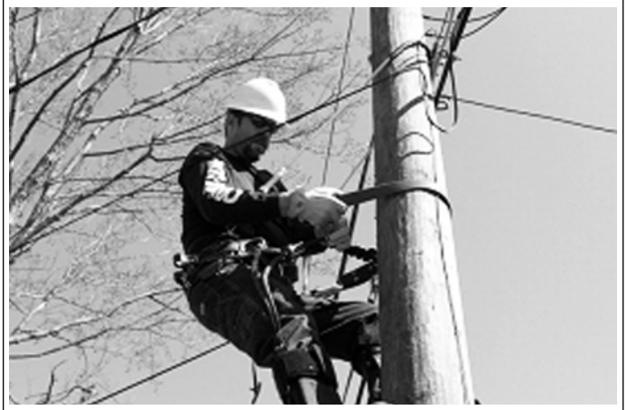
Figure 31 - Reconnect Strap or Lanyard
