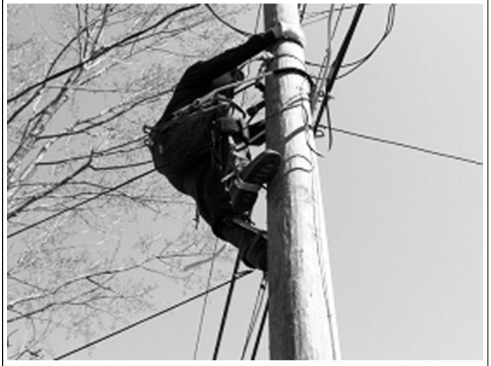
Figure 31 - Reconnect Strap or Lanyard
