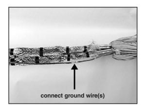
4.10 Unfold the cable fillers and reestablish their lay between the cable conductors. Hold the fillers in place with a band of Scotch® Super 33+ Vinyl Tape.
