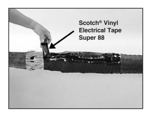
6.5 Apply two half-lapped layers of 4" wide 3M™ Scotch-Seal™ Mastic Tape 2229 over applied vinyl tape in splice center. Overlap ends of Cold Shrink jacket tubes 2" (51 mm).
