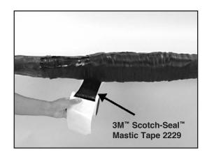
6.6 Cover the applied 3M<sup>™</sup> Scotch-Seal<sup>™</sup> Mastic Tape 2229 with two half lapped layers of Scotch<sup>®</sup> Vinyl Electrical Tape Super 88.
