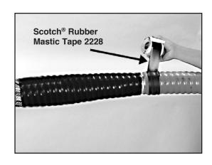
6.3 Install a cold shrink jacket tube on each cable with the leading end just covering the Scotch® Rubber Mastic Tape 2228 and the tube extending toward the splice bodies.
