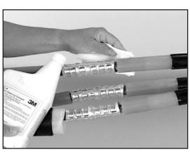
4.5 Apply red compound on cable insulation, making certain to fill in edges of cable semi-con.
