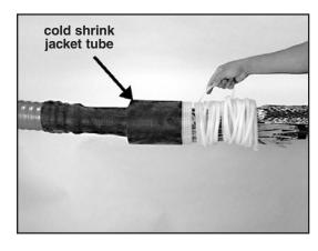
6.4 Apply one half lapped layer of Scotch® Vinyl Electrical Tape Super 88 over the unjacketed area in splice center.
