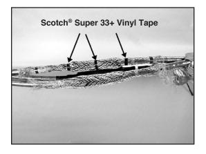
4.8 Connect sleeve ends to the cable metallic shield with a small constant force spring.
