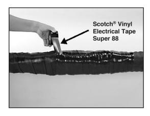
6.7 Overwrap the entire splice with a minimum of two half lapped layers of 3M<sup>™</sup> Sheath Wrap.
