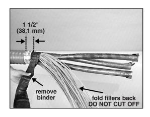
2.3 Cut the phase conductors to the appropriate length.
