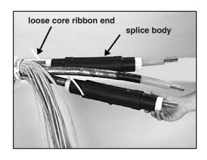
3.3 Expand metallic shield sleeves and slide one onto each conductor of **Cable Y**. Compress the ends of each shield sleeve together next to the cable armor or jacket end, away from the prepared conductor ends.
