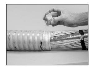
5.2 Wrap an end of the ground continuity braid around exposed armor and applied Scotch® Electrical Shielding Tape 24 on one cable end.
