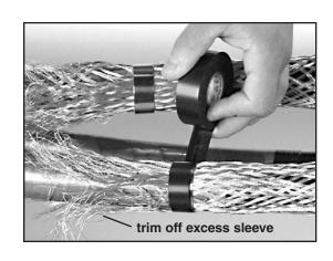
4.9 Connect the ground wire(s) from **Cable X** to the ground wire(s) from **Cable Y**. Make the connection away from the splice bodies.
