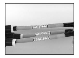
4.2 Apply a tape marker to cable semi-con insulation shields on Cable Y (cable side which does not contain splice body) at a distance of 9"
