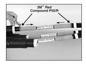
4.6 Individually, position each splice body over the connector area and align the leading end of the rubber with the center of the marker tape.
