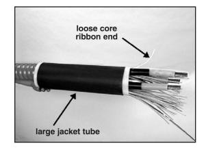
3.2 Slide a cold shrink splice body onto each conductor of **Cable X** with the loose core ribbon end going on the cable first, away from cable end.
