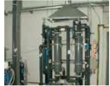
3M™ Liqui-Cel™ Water Degassing System used at the Ice Palace to produce crystal clear ice at the arena
