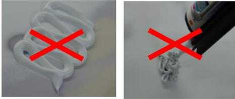
To prevent air entrapment, avoid applying material as shown (no spaghetti balls / spaced bead)
