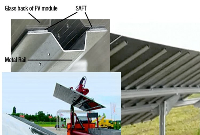
Figure 1. Dual-Glass PV Solar Panels mounted with 3M SAFT.
