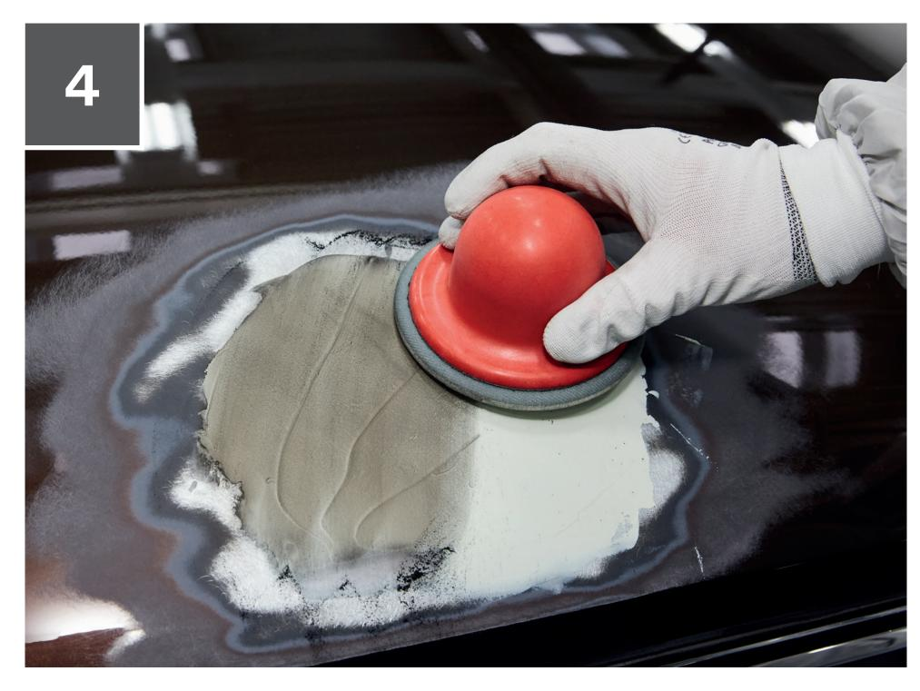
Apply 3M<sup>™</sup> Dry Guide Coat and hand or machine sand the filler to the desired shape.
