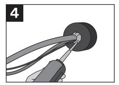
Fill all voids and interstices of cables with  $3M^{\text{\tiny M}}$  Fire Barrier Rated Foam FIP 1-Step, full depth of the plug.
