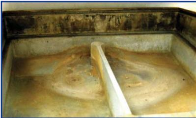
Without filtration, impurities in water can result in increased build up resulting in increased maintenance and the possibility of reduced equipment life.
