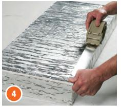
All corners and butted seams in the mat are to be covered with minimum 2 mil aluminum foil tape.
