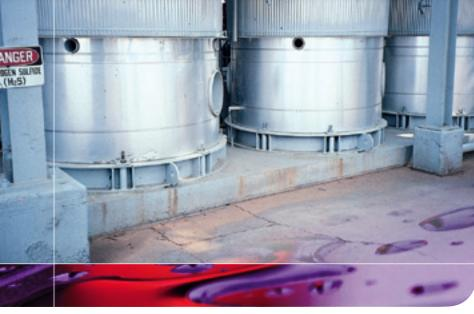
When 3M<sup>™</sup> Interam<sup>™</sup> Endothermic Mat is applied to vessel skirts and pipe lines, it minimizes the effects of fire exposure by flame impingement in order to reduce the steel's rate of temperature rise and to delay structural failure.
