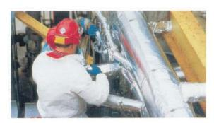
Installing the ceramic mat insulation on the complex conduit lines at Ashland's St. Paul plant was hastened by the ability to cut and fit the material with common tools
