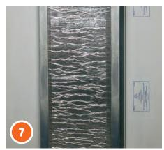
View of the protected box from the backside prior to installing the gypsum wallboard.
