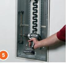
Insert the utility box into the opening so the box is flush with the surface of the wall. Secure the steel box to the steel studs per the utility box manufacturer's installation instructions.
