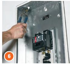
The bottom or top of the steel box may be penetrated by up to 2" metallic conduit. See system parameters.
