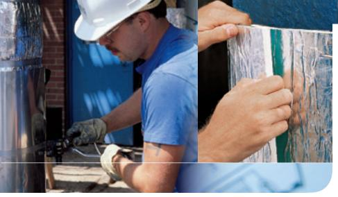
Installing multiple layers of 3M<sup>™</sup> Interam<sup>™</sup> Endothermic Mat flexible wrap allows you to tailor the desired amount of fire protection—up to 4 hours for structural steel.
