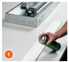
Cut the 3M<sup>™</sup> Interam<sup>™</sup> Endothermic Mat to fit the sides, top, bottom and back of the utility box. Apply 3M<sup>™</sup> Super 77 Multipurpose Adhesive to the box surface and each piece of mat. Let the adhesive dry on the box and mat surface for approximately 1 minute. See UL System W-L-7190 for overlaps and complete system details.
