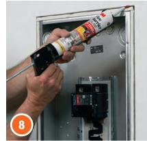
Apply a nominal 1/4" diameter bead of sealant at the mat and gypsum interface.
