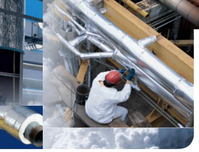
3M<sup>™</sup> Interam<sup>™</sup> Endothermic Mat is designed to provide cable trays and conduits with full envelope protection in the event of a fire.
