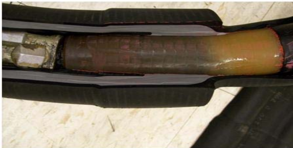
Figure 2. Sample A Inspection of Connector and Cable Insulation After Load Cycling
