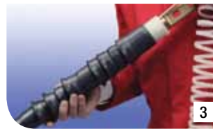
3 Begin to remove the inner core, allowing the termination to shrink down onto the cable
