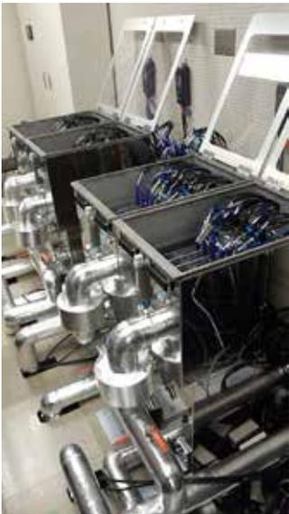
The Suiren, a supercomputer developed by PEZY Computing and ExaScaler Inc., is cooled by a single-phase immersion cooling system, the ESLC-8 Submersion Cooling system, using 3M™ Fluorinert™ Electronic Liquid as the heat transfer medium.
