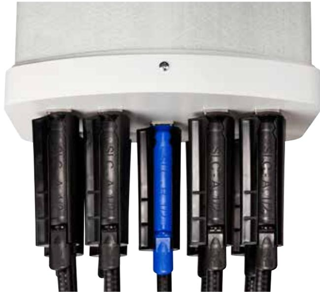
3M™ Slim Lock Closures installed on an antenna
