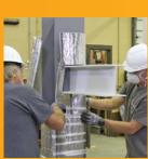
Installing multiple layers of 3M™ Interam™ Endothermic Mat E-5A-4 flexible wrap allows you to tailor the desired amount of fire protection—up to 4 hours for structural steel.
