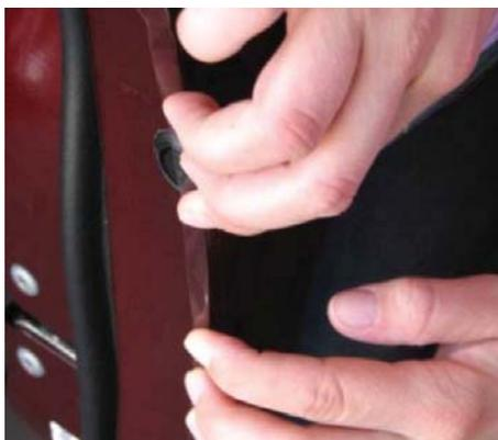
8. After starting to secure the edge, continue to fold the film around to the back of the door edge over the entire length of the door.
