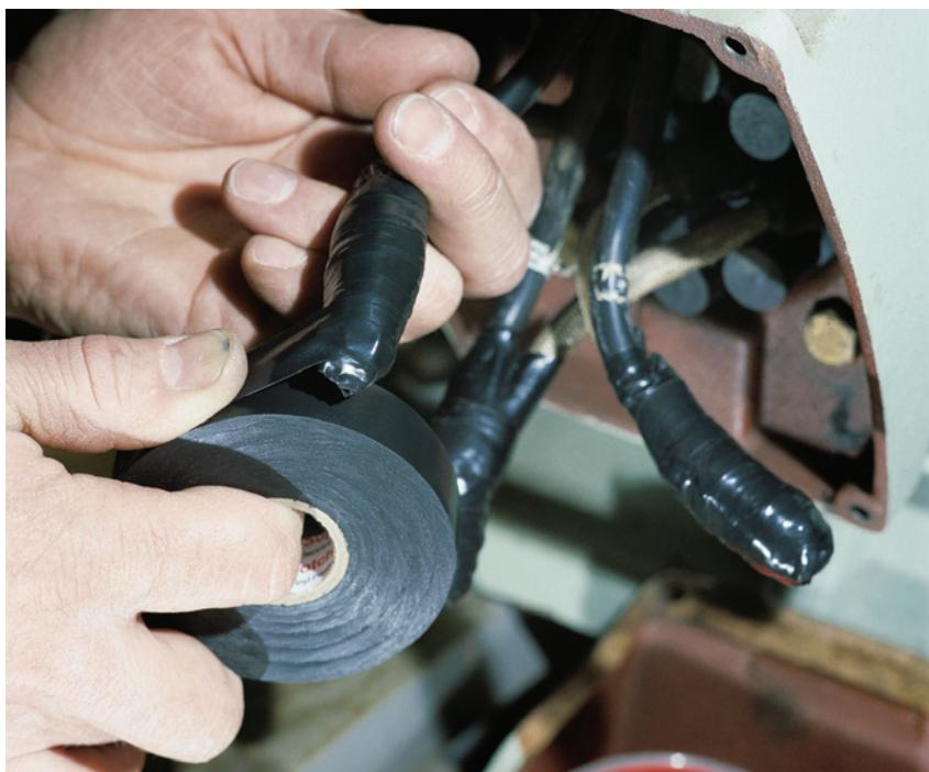
Three different types of tape are used to connect feeder cables to motor leads. In the last step, a quality vinyl electrical tape is stretched as it is wrapped for good conformance to the underlying structure and to complete the moisture seal. This tape withstands the effects of vibration while providing electrical insulation and protective jacketing.
