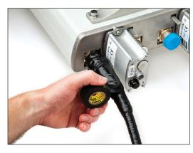
4.9 Wrap three (3) half-lapped layers of ¾" (19 mm) vinyl tape starting 1" (25 mm) beyond the previous layer of vinyl tape, up to the base of the antenna.
