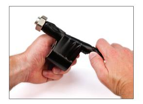
4.4 Starting 1" (25 mm) below the previous vinyl tape layer, wrap the cable with three continuous half-lapped layers of ¾" (19 mm) wide 3M™ Temflex™ Vinyl Electrical Tape 1700 up to the connector clamping nut.
