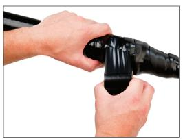
2.7 Finally, wrap the entire section of cable with three continuous half-lapped layers of ¾" (19 mm) wide vinyl tape. Begin and end the final three layers 1" (25 mm) beyond each end of the previous layer of vinyl tape.
