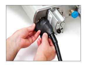
4.8 Wrap two (2) half-lapped layers of 2" (51 mm) vinyl tape starting 1" (25 mm) beyond the butyl mastic tape and up to the base of the antenna.
