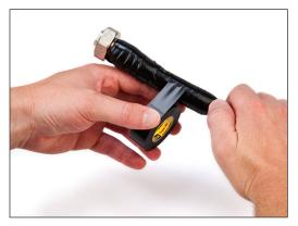
4.5 Connect the jumper cable to the antenna connector to the proper torque specification.
