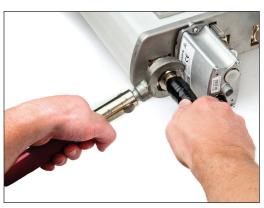
4.6 Start 1" (25 mm) below the connector clamping nut and apply one (1) half-lapped layer of ¾" (19 mm) vinyl tape extending 1" (25 mm) beyond the cable connector clamping nut. Wrap up to, but short of, the base of the antenna. If space restrictions prevent wrapping tape from roll, then the tape can be applied in one (1) or more strips if necessary, or a strip can be wound onto a small applicator, (e.g. a pencil), and unwound around the connection assembly.
