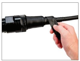
2.5 Once smooth tapered transition is complete, use butyl mastic tape to create environmental seal. Start 2" (51 mm) beyond the first layer of vinyl tape and make half-lapped layers extending 2" (51 mm) past the opposite end of the first layer of vinyl tape. Smooth by hand.
