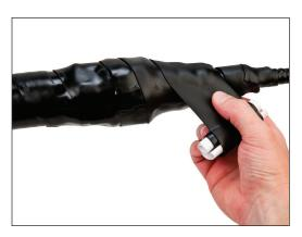
2.6 Next, beginning 1" (25 mm) beyond the layer of butyl mastic tape applied in step 2.5, wrap the entire section of cable with one or two layers of half-lapped 2" (51 mm) Scotch® Vinyl Electrical Tape 700 extending 1" (25 mm) beyond the layer of butyl mastic tape.
