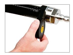
2.4 Using the butyl mastic tape, build up the jumper cable diameter near the feeder cable to create a smooth tapered transition. (To create taper, strips of butyl tape may be folded in half lengthwise for faster build up.) Taper should end at the same point as the first layer of vinyl tape. Smooth final layer by hand.
