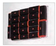
12.4 The smaller-sized self-locking pillows are useful for smaller voids and spaces created by the cable tray. 3M™ Moldable Putty+ is used to seal any small openings greater than 1/16" (1.59 mm) between the pillows, cables, cable trays and pillows within the frame.
