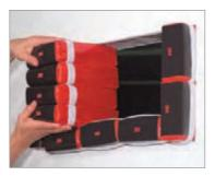
12.3 Completely fill the penetration opening. The red 3M logo must be visible to the installer on all pillows.
