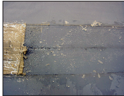
Polyurethane Protective Tape Removal
