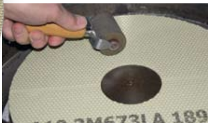
5. Roller over the entire surface paying particular attention to the edges.
