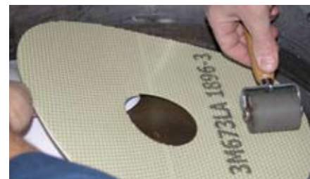
4. Roller with even pressure and pull the liner back.
