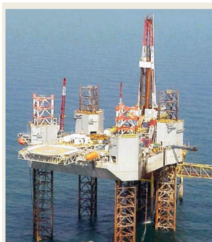
Fig. 1. The independent-leg cantilever jackup GSF Britannia is one of 23 rigs owned by GlobalSantaFe that used ozone-depleting halon fire-protection systems.
