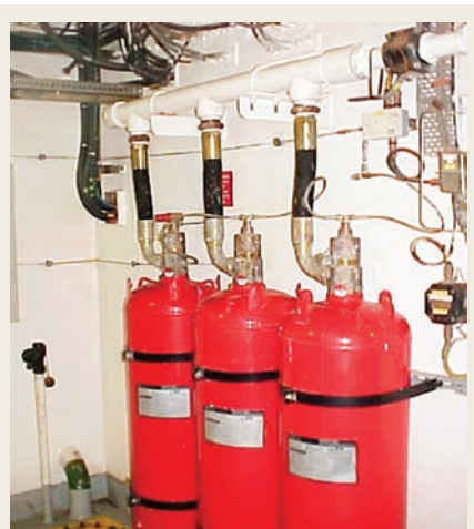
Fig. 2. On the GSF Britannia and other rigs in its fleet, GlobalSantaFe has begun phasing out its halon fire extinguishers in favor of the non-ozone-depleting alternative.
