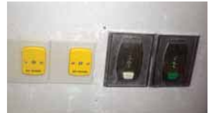
3M™ Interam™ Endothermic Mat meets the stringent requirements of firestopping for wall-mounted medical gas access cabinets commonly found in hospital patient rooms.
