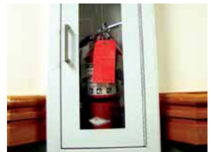
A single layer of 3M™ Interam™ Endothermic Mat material on fire extinguisher boxes meet the International Building Code for a one-hour fire barrier.
