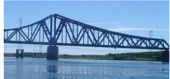
The CTEEP 138 kV Line Runs Parallel to a Railroad Bridge
