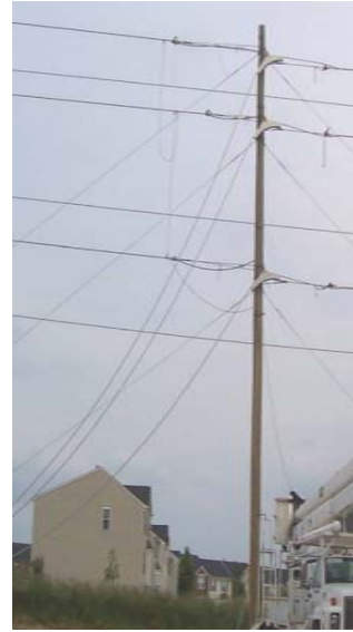
Temporary pole, roller arrays and conductor, Tower 3
