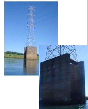
Concrete Foundations, the Paraná River Crossing, Brazil
