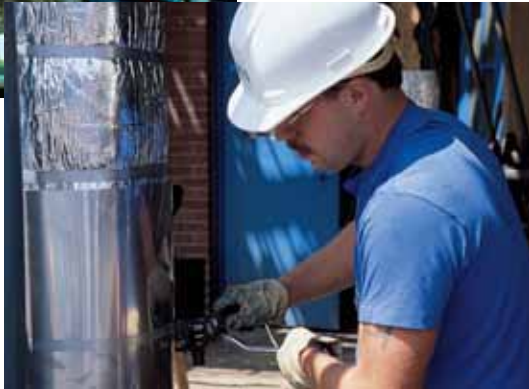
Multiple layers of 3M™ Interam™ E-Mat Flexible Wrap allow you to tailor the exact amount of fire protection you desire.
