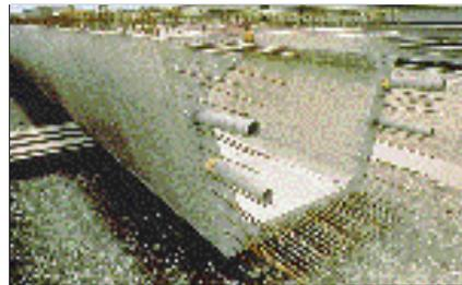
Fig. 5 Section of pre-stressed concrete. Metal bars are in tension, concrete is in compression.
