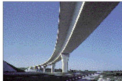
Fig. 4 Pre-stressed concrete bridge span. The beam is subject to bending moments which generate tensile stresses.
