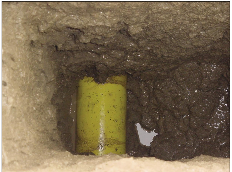
Once the pipeline was exposed, workers measured the depth from grade to pipeline (Fig. 3)
