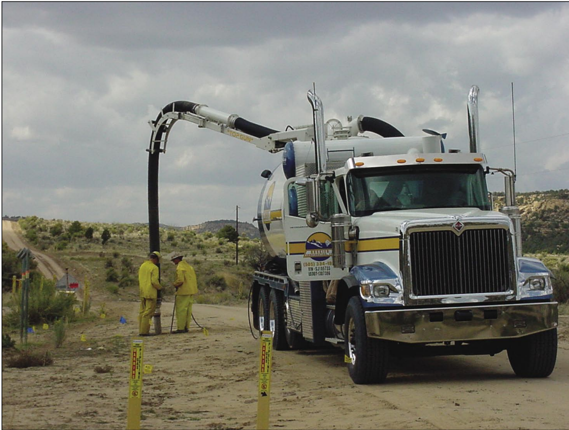
BP excavated each rural road crossing in its New Mexico region to expose buried pipeline (Fig. 2).
