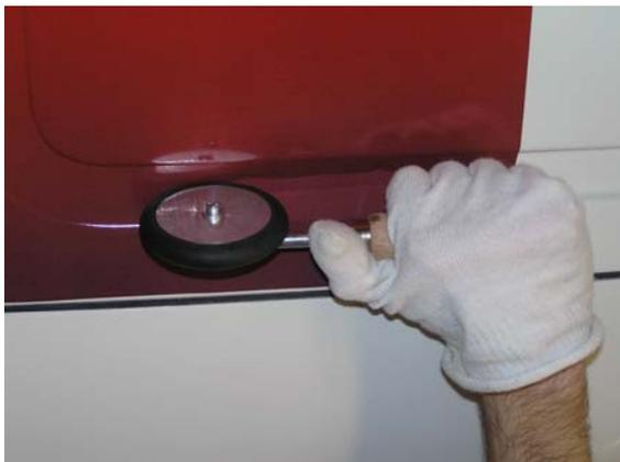
11. Using manual application or the hand-roller, heat the film to a temperature of approximately 50°C and continue applying the film to the flat part of the recess until a small air channel remains between the film and the corner of the recess.
