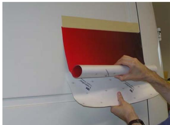
5. Start the application on the flat part of the substrate and bridge the film over the recessed areas and deep corrugations. Use a Gold PA-1 applicator to apply the film on to the substrate. Avoid air entrapment between the film and the substrate. If the graphic does not use application tape, use a 3M Cotton Squeegee Sleeve\* on the PA-1 applicator.
