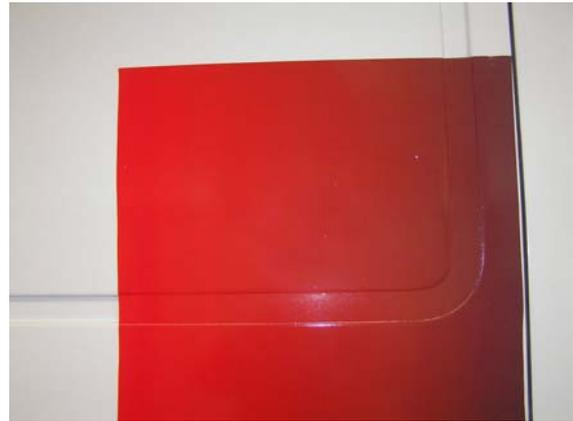
8. Stretch the film into the centre of the recess starting from the middle working towards the edges of the film.
