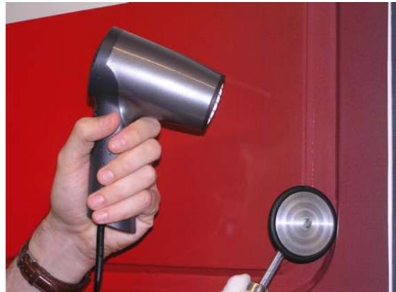
13. Air bubbles between the film and the substrate must be removed with the air release tool.
