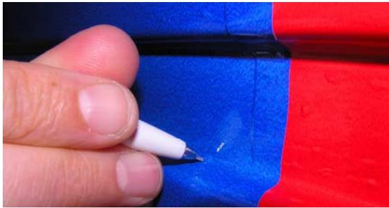
16. Remove the detected air bubbles with the air release tool.
