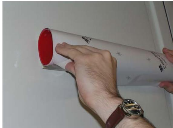
4. Remove the liner carefully from the film.
