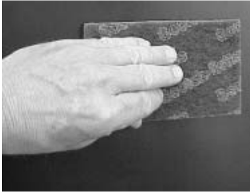
Figure 5. Scuffing Wall to Enhance Film Adhesion
