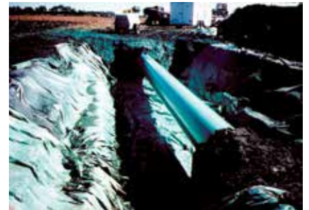
Completed pipe coating rehabilitation using 3M™ Scotchkote™ Liquid Epoxy Coating.
