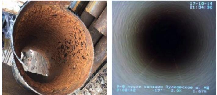
Twenty-four inch steel pipe in St. Petersburg, Russia, before and after lining with 3M™ Scotchkote™ Pipe Renewal Liner 2400.
