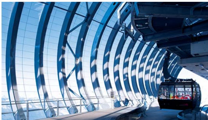
Fig. 7: The façade of the mountain station of the glacier cable car on the Gaislachkogel, Austria. ETFE films (Nowoflon ET 6235Z) are used and have been designed to withstand extreme wind loads, high UV levels and low temperatures. (Copyright: A. Niederstrasser)
