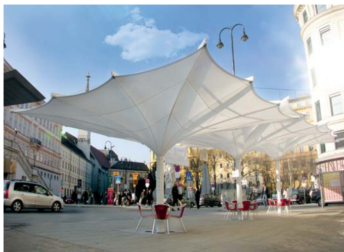
Fig. 1: The sun protection sails covering the Café Mozart in Vienna, Austria, are made from a yellowing-resistant, translucent PTFE fabric.
