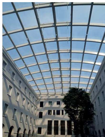
Fig. 3: The inner courtyard of the William Rappard Centre of the World Trade Organisation in Geneva, Switzerland, is spanned by Nowoflon ET 6235Z films made from ETFE. Plants and trees can grow under this self-cleaning, transparent construction. (Copyright: WTO)
