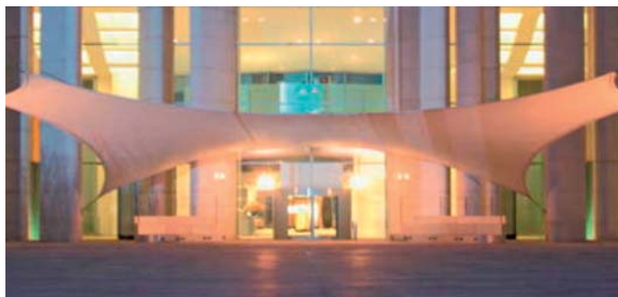
Fig. 4: The entrance to the Federal Chancellor's Office in Berlin, Germany, is probably one of the most photographed fluoroplastics applications. The construction consists of a PTFE-coated glass fibre fabric.
