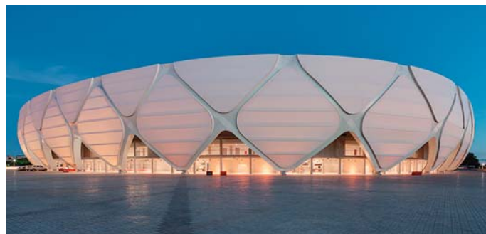
Fig. 5: Sports stadia – here the Manaus Stadium in Brazil shows a popular application for fluorothermoplastic films. (Copyright: M. Bredt)
