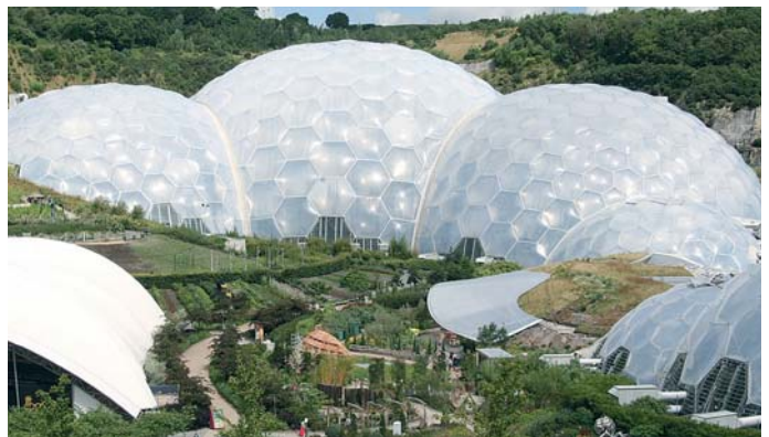
Fig. 8: The "biomes" at the Eden Project in Cornwall, UK, consist of a cushion construction made using ETFE. Films made from Dyneon ETFE let pass 90 % of the visible light and 80 % of the UV-A light.
