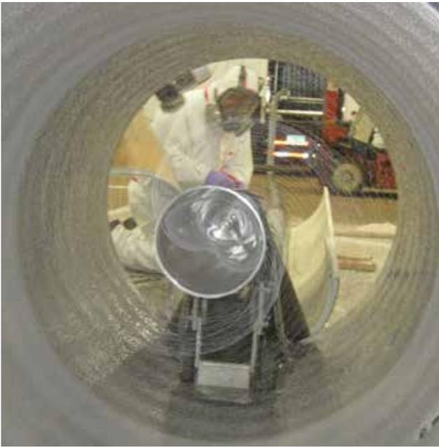
Lining a 36-inch Pipe with 3M™ Scotchkote™ Pipe Liner 2400 in the 3M Lab
