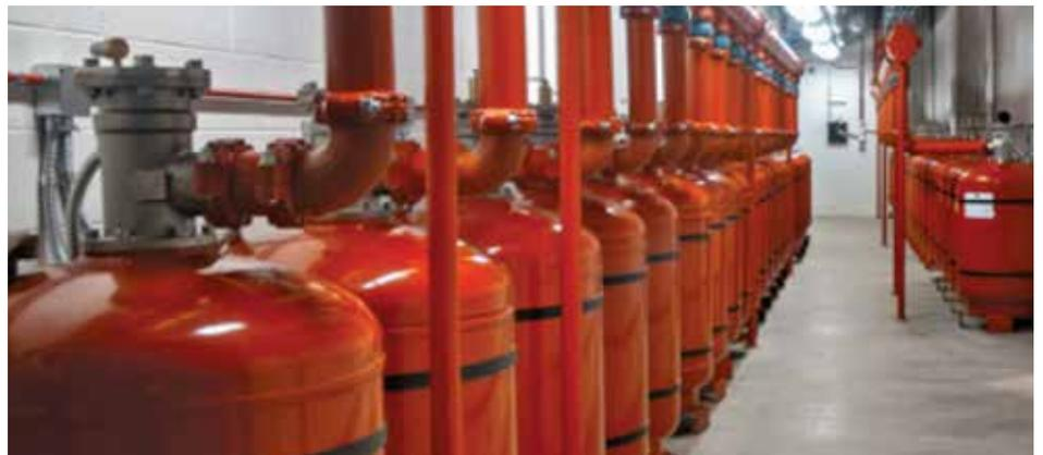
3M™ Novec™ 1230 Fire Protection Fluid is engineered as a more sustainable alternative to legacy first-generation halon replacements such as HFCs. Its unique properties also allow safe system design at higher pressures.
